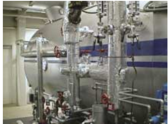
Heat insulation of boiler piping
