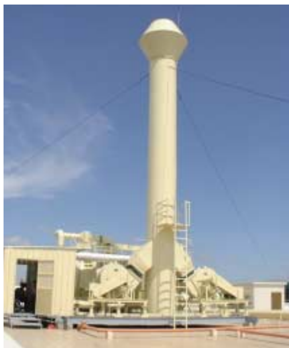
Newly installed emission control facilities
