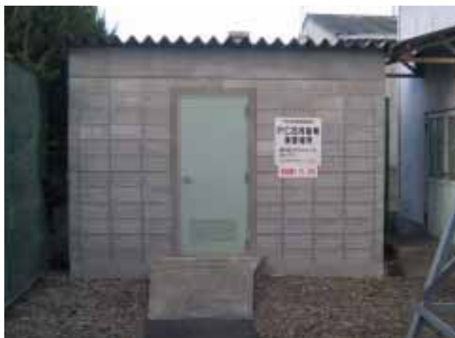
State of PCB storage
