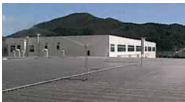
Energy-saving using sprinklers
